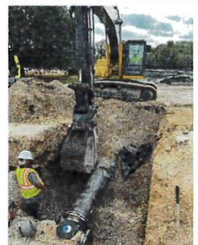
Figure 4: Relocating yard piping at UG-03 per RFI005A.
