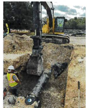
Figure 4: Relocating yard piping at UG-03 per RFI005A.
