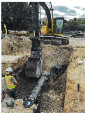
Figure 4: Relocating yard piping at UG-03 per RFI005A.
