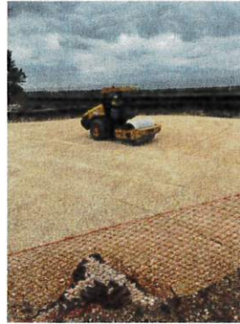
Figure 3: Compacting lift #9 of the GST select fill material.
