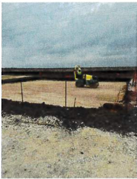
Figure 1: Select fill compaction at the pump station building.
